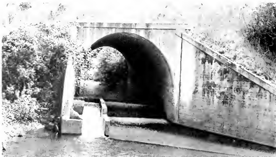
FIG. 36. Rattlesnake Creek, with drop inside the arch culvert. Note fish ladder at left
